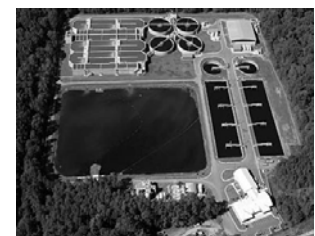
Durham County North Carolina WWTP
